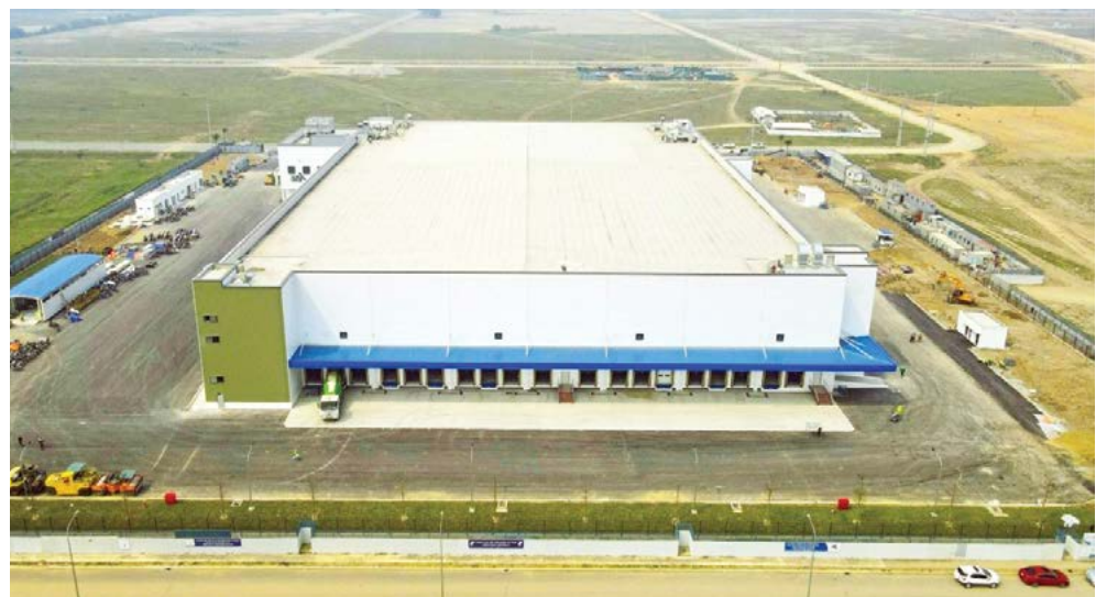
Yen Phong Industrial Park 2c
